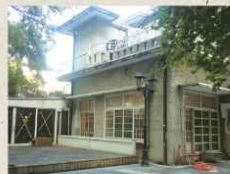
▲ Figure 20 – Before restoration, 2018
