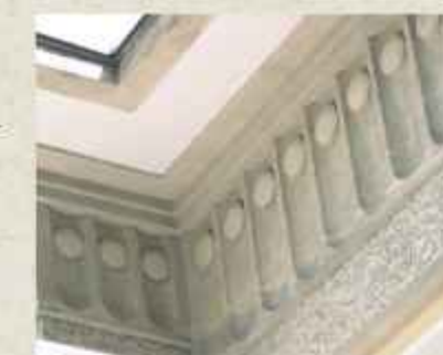
▲ Figure 5 – Eaves of the brick structure, ornamented with circles and ovals
