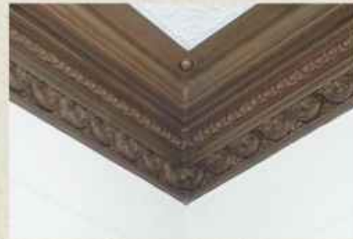
▲ Figure 17 – Egg-and-dart cornice, main hall
