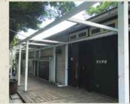
▲ Figure 18 – Before restoration, 2018
